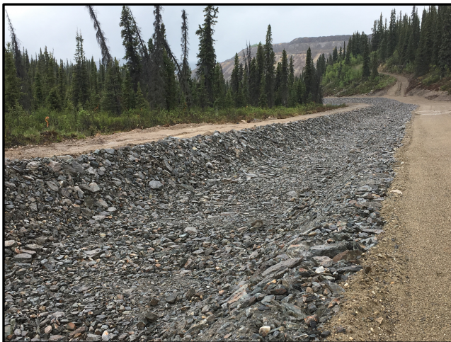
Figure 2. Faro Mine, North Fork Rose Creek Diversion Channel, June 2019
